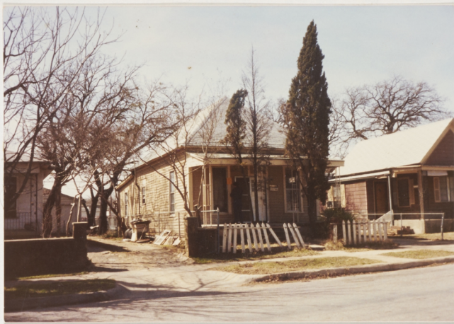
Marine Schoolhouse Winter 1989 Before it was boarded up
