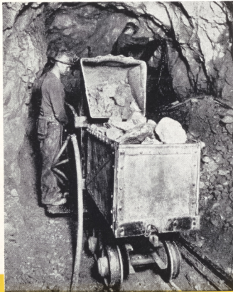
Same loader discharging into car. Note how completely and evenly the car is filled. Note, also, large size of bucket (six cubic feet) which enables average operator to load a 20-cubic foot car in less than one minute at moderate working speed. Our Model 20 machine is equally effective for loading larger cars.
