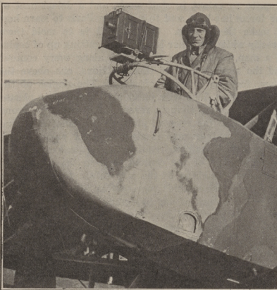
THE AIR CAMERA IS FLEXIBLY MOUNTED
